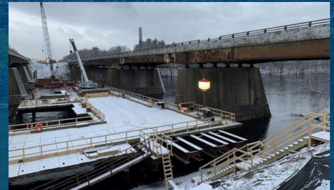
Example of a temporary trestle used for construction
